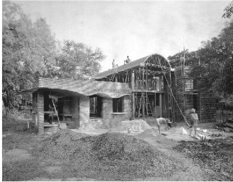
Building a new house
