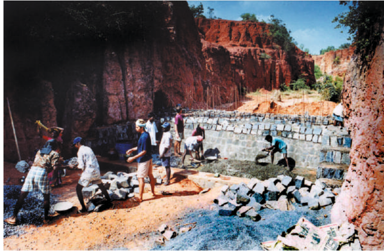
Check dam building
