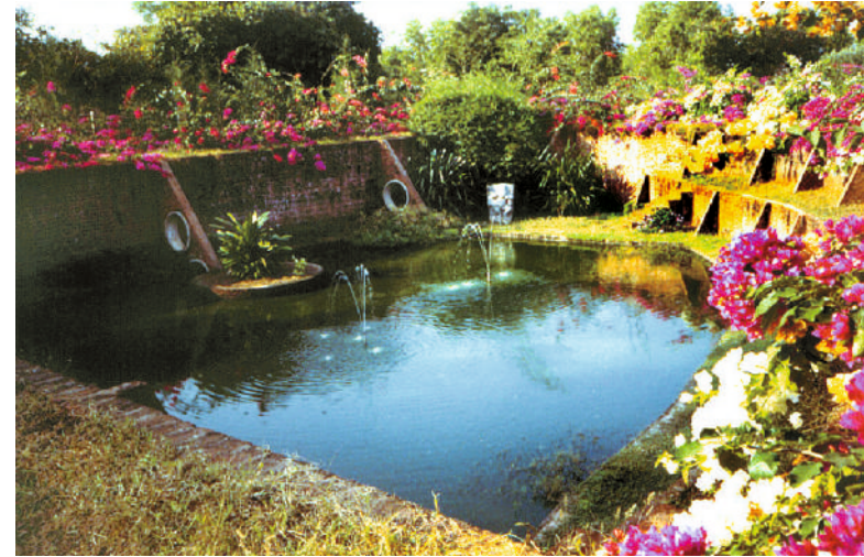
Waste water treatment plant
