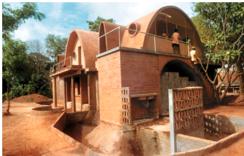
Earth block construction
